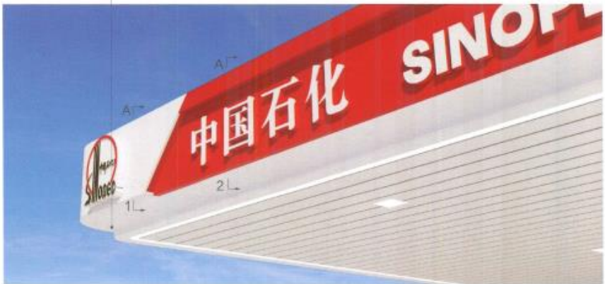
Eaves lower cladding panel (1.5mm thick white aluminum sheet)
